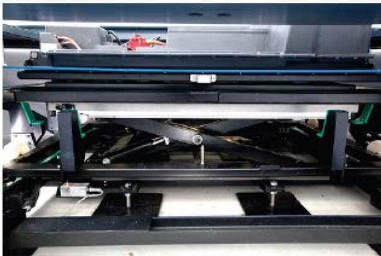
BSS Battery Switch In-Progress
